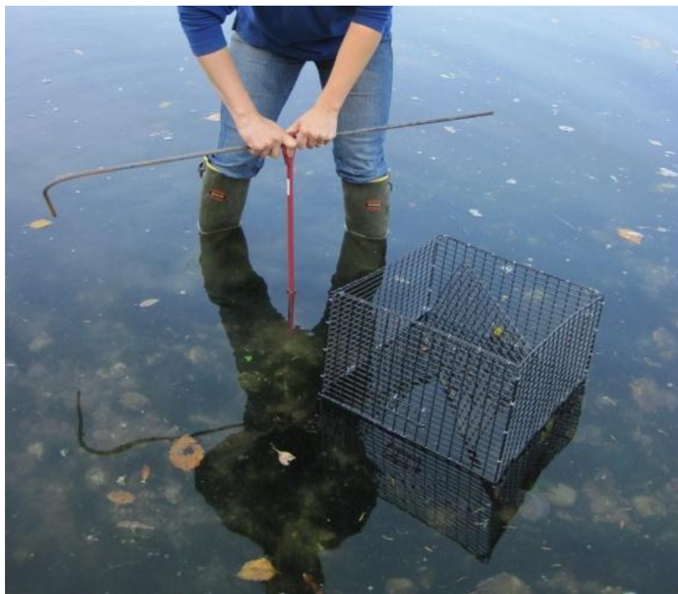
Figure 2 Screwing in 76.2 cm (30 inch) screw anchor.
