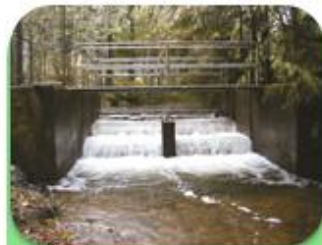
Fish Passage Correction
