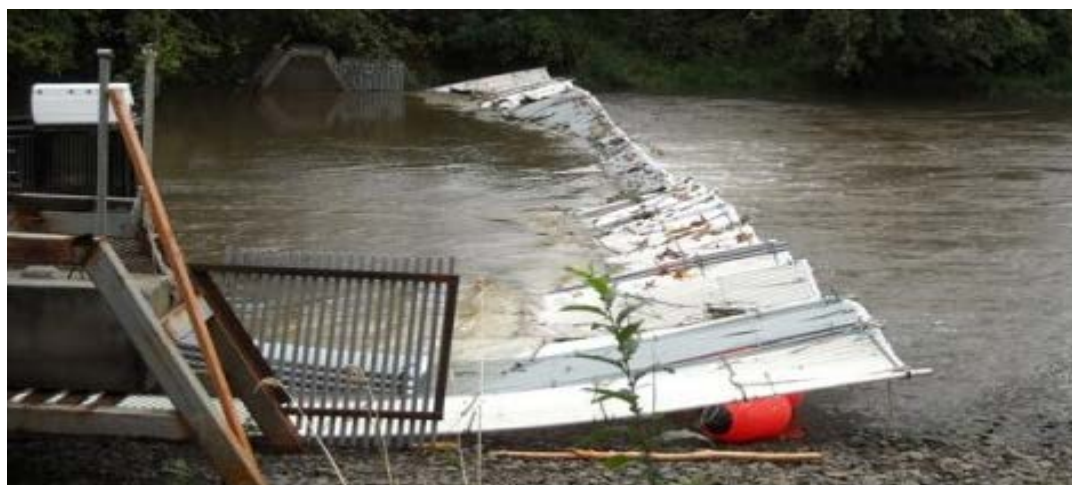
Figure 3. 2010 Grays River Weir configuration. Photo credit: Jeremy Wilson (WDFW).
