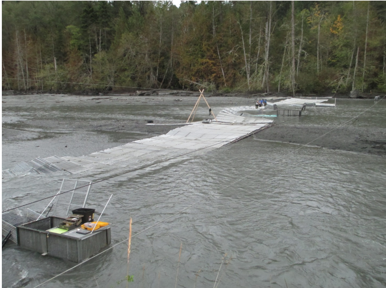
Figure 6. Elwha weir site during summer 2013 trapping period. The left bank channel (approximately 40% of flow) is in the foreground and right bank channel (approximately 60% of flow) is in the background. Note exposed central gravel bar mid-channel. Photo taken Aug 15, discharge = 750 cfs (USGS gage 12045500).
