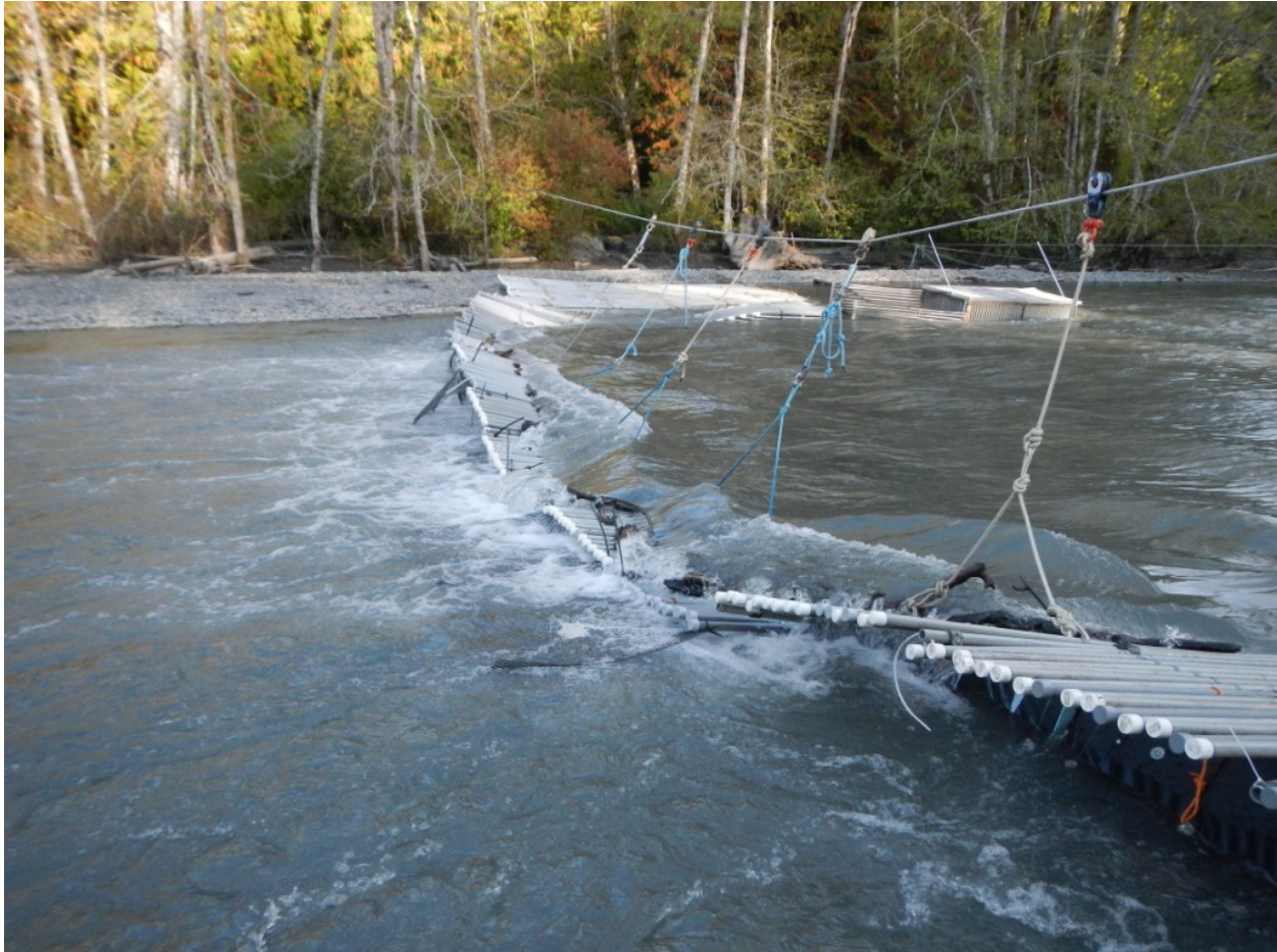
Figure 7. Weir panels with bridles and winged resistance boards, partially sunk from debris loading. Photo taken Aug 13 2013, discharge = 652 cfs (USGS gage 12045500), from central gravel bar looking towards right bank channel.
