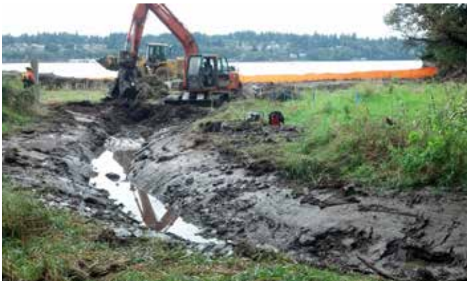
Mission Creek during excavation
