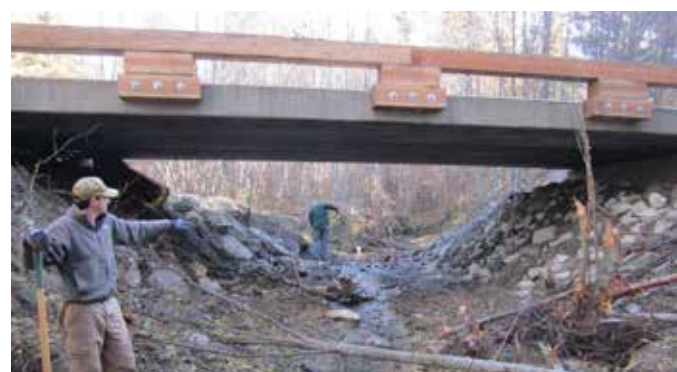
East Fork Tunk Creek fish passage project (before and after)
