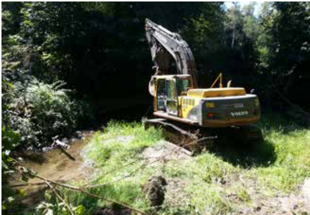
Gorst Creek Floodplain, 1st day of construction
