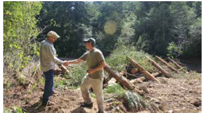
Engineer and construction contractor of Clearwater log jam
