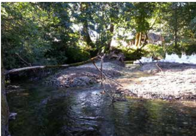
Gorst Creek Floodplain & mid-channel Apex Jam after construction
