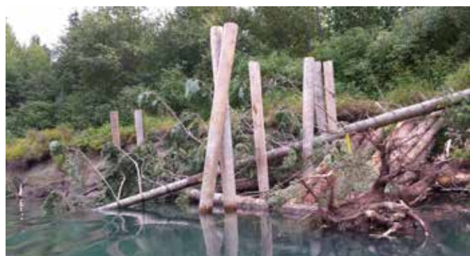
White River Large Wood Atonement (under construction)
