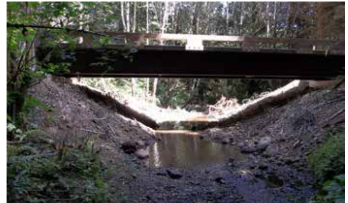
Coal Creek bridge after construction
