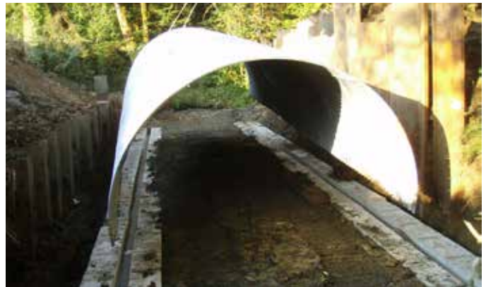
Installation of new culvert in Cedar Creek
