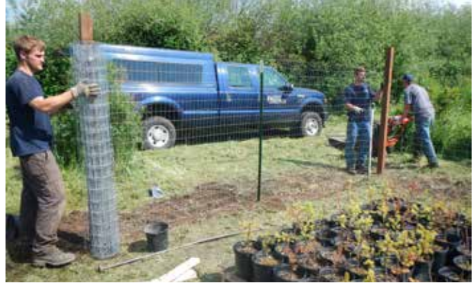
WCC crew installs a deer fence around the NOSC native plant nursery.
