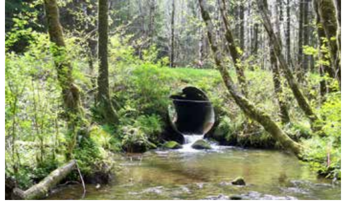
Coal Creek plunge pool before construction
