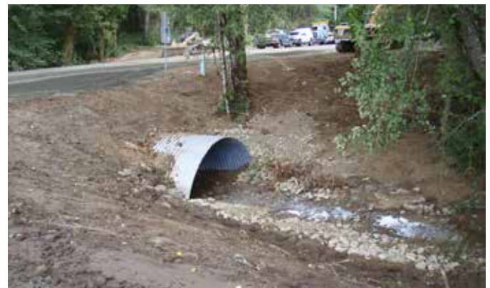
Completed Cedar Creek project
