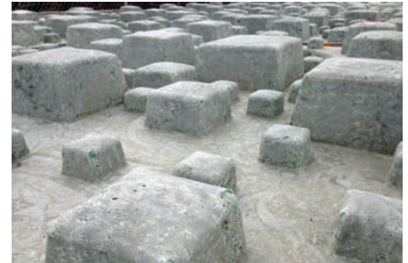
Roughness panels will help improve fish passage
