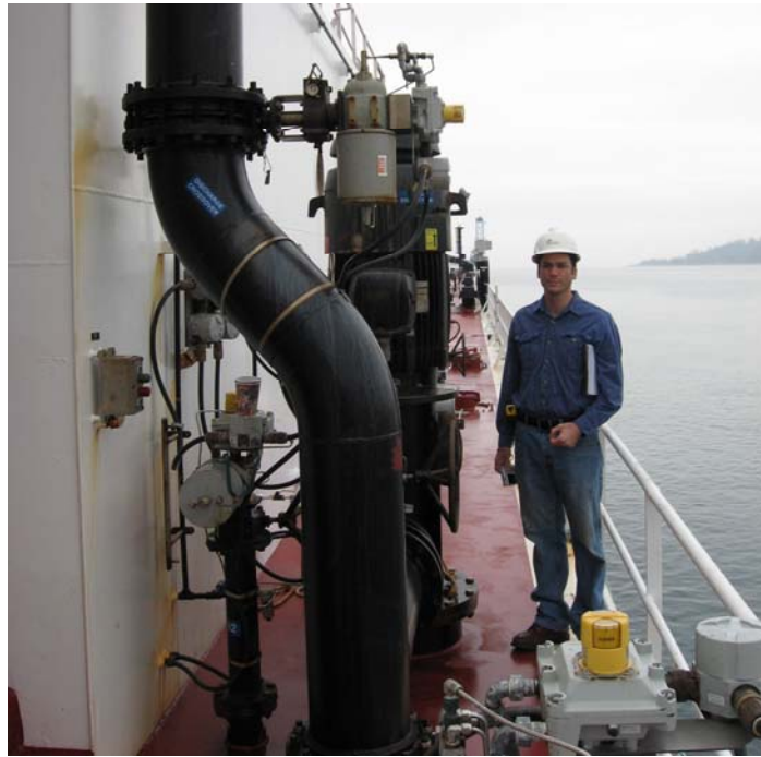
Figure A-2. Deck Side
