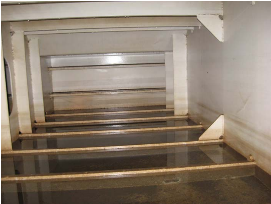
Figure A-12. Inboard, double bottom portion.
