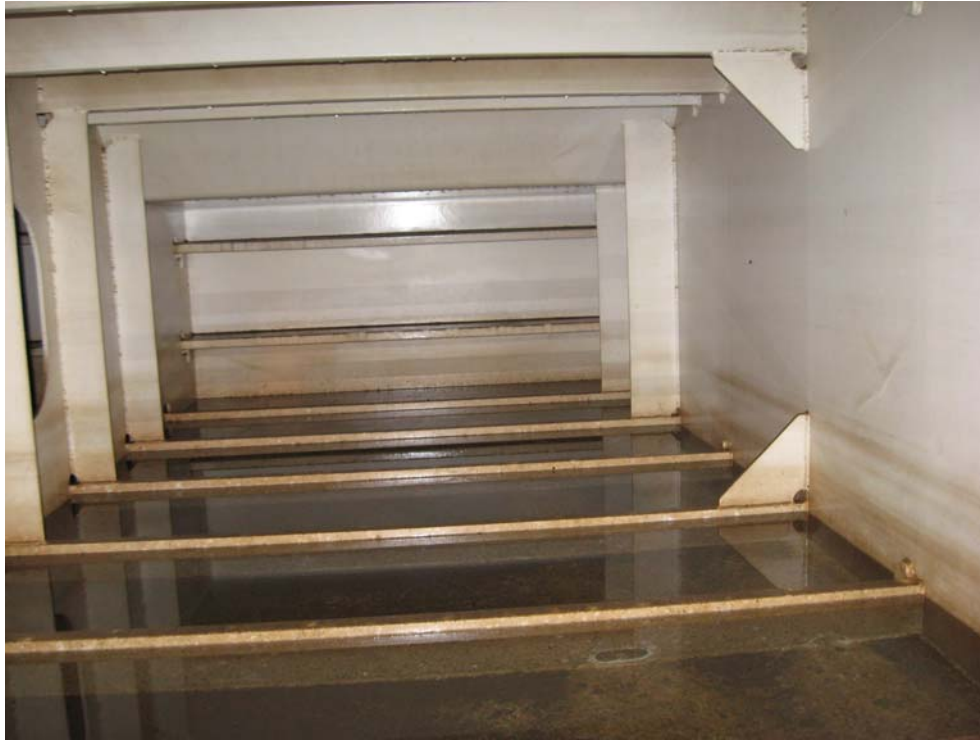
Figure B-3. Double bottom portion of the ballast tank.
