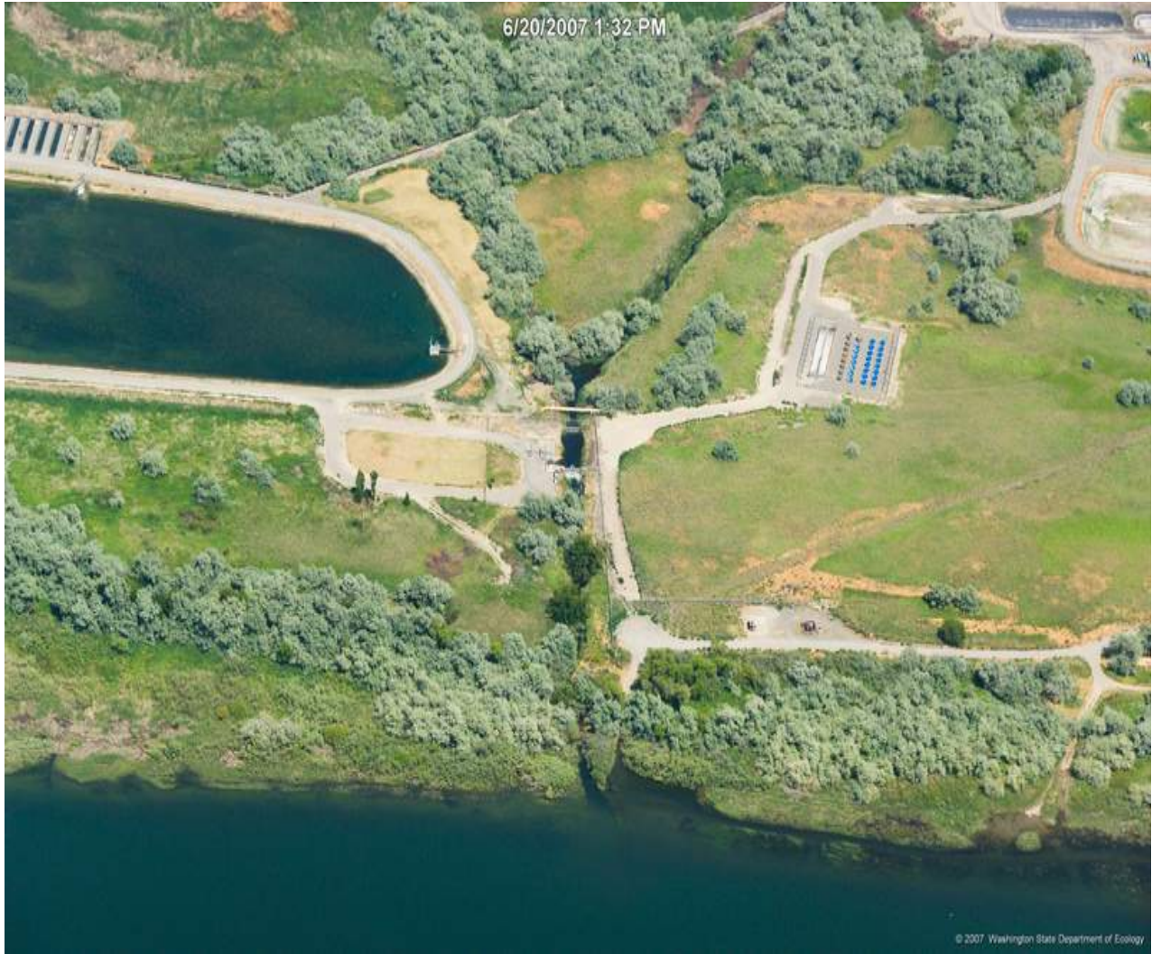
Figure 3. RSRF 9-acre pond, outlet structure, fish trap, 2 concrete raceways and 32 blue round tanks.
