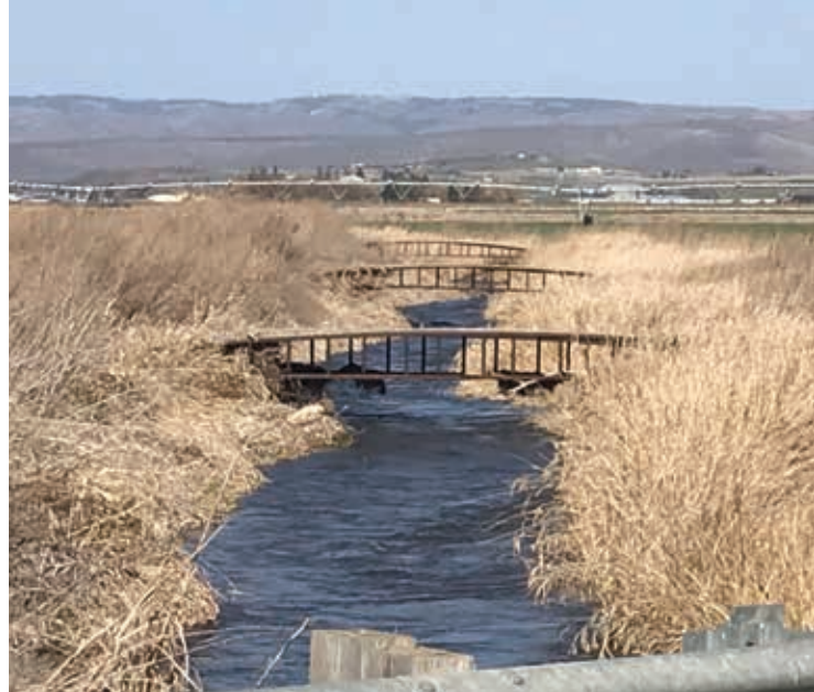
A modified riparian area within an agricultural landscape in Kittitas County. The stream channel was likely straightened decades ago. More recently, small bridges were built across the stream for pivot sprinklers to move back and forth. To allow ease of sprinkler movement, no woody vegetation is allowed to grow./Jennifer Nelson, WDFW
