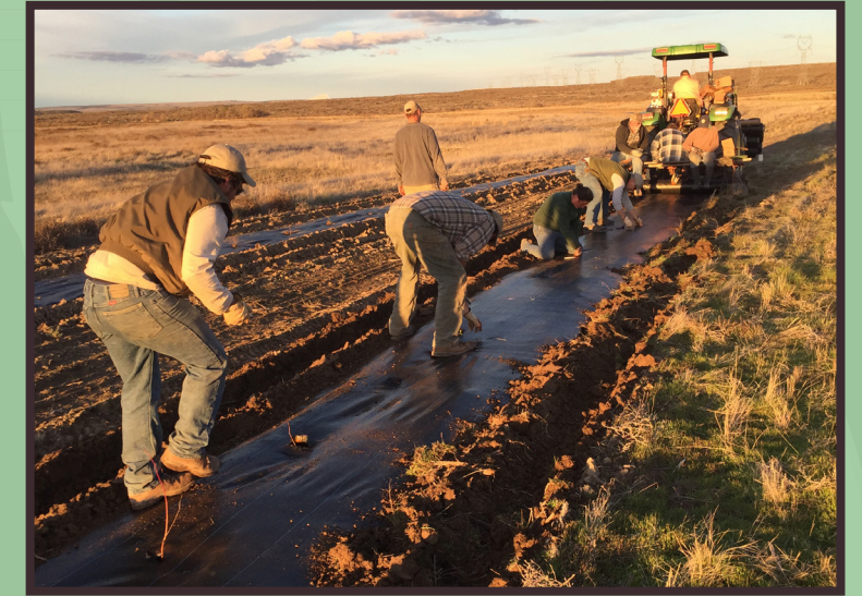
Stream Bank Stabilization and Nesting Cover
