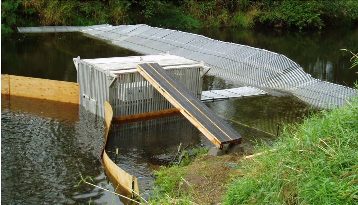
Figure 6. Coweeman River Weir configuration. Photo credit: Patrick Hulett (WDFW).
