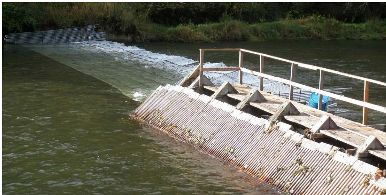
Figure 8. Green River Weir configuration. Photo credit: Amanda Danielson (WDFW).
