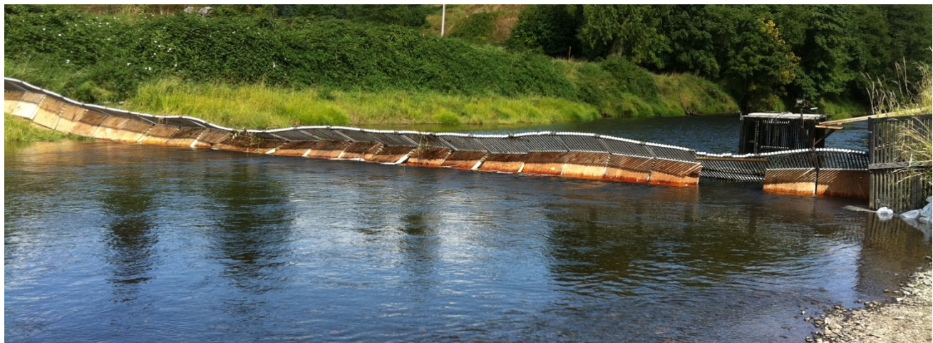
Figure 3. Grays River Weir configuration.
