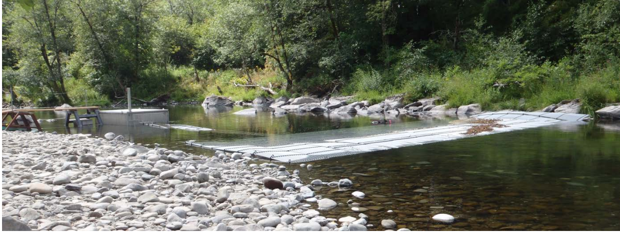
Figure 10. Washougal River weir configuration. Photo credit: Eric Kinne (WDFW).
