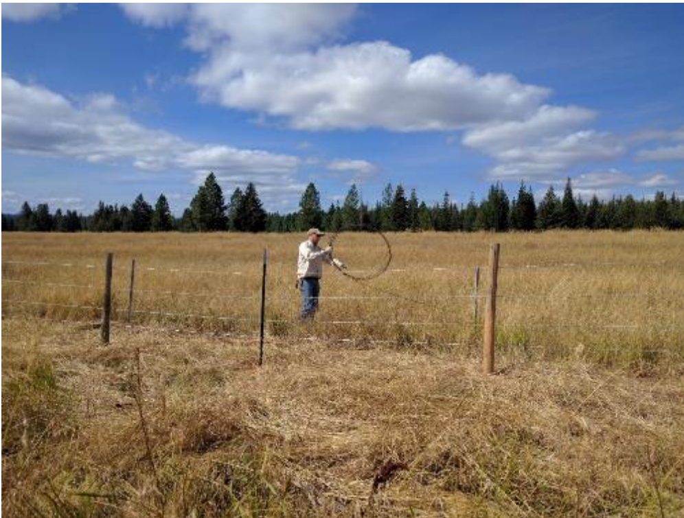
Fence Work on the 4-O Ranch Unit (Patricia Jatczak)
