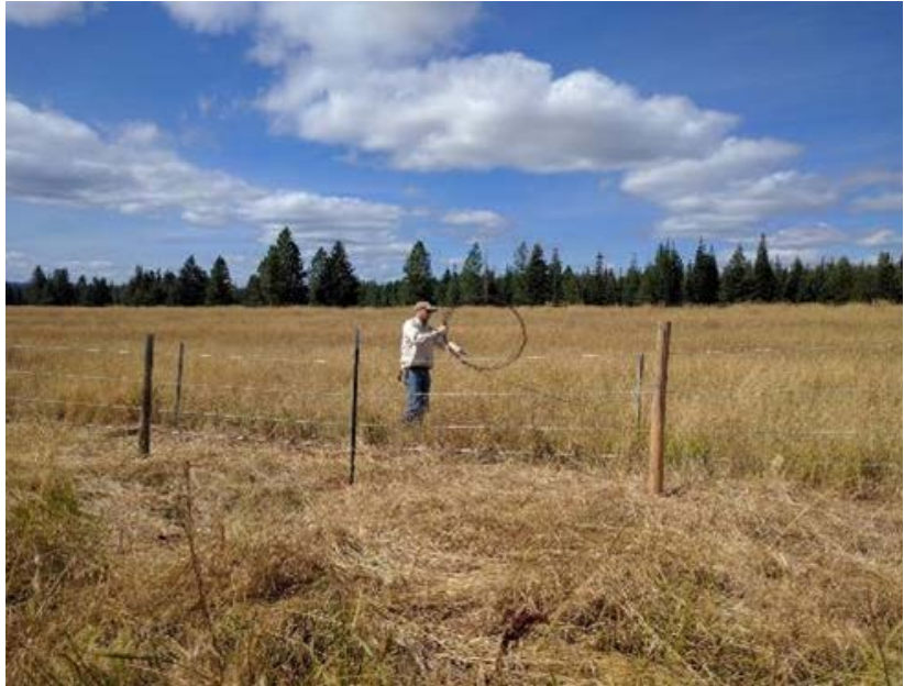
Fence work on the Grouse Flats Unit Photo by WDFW
