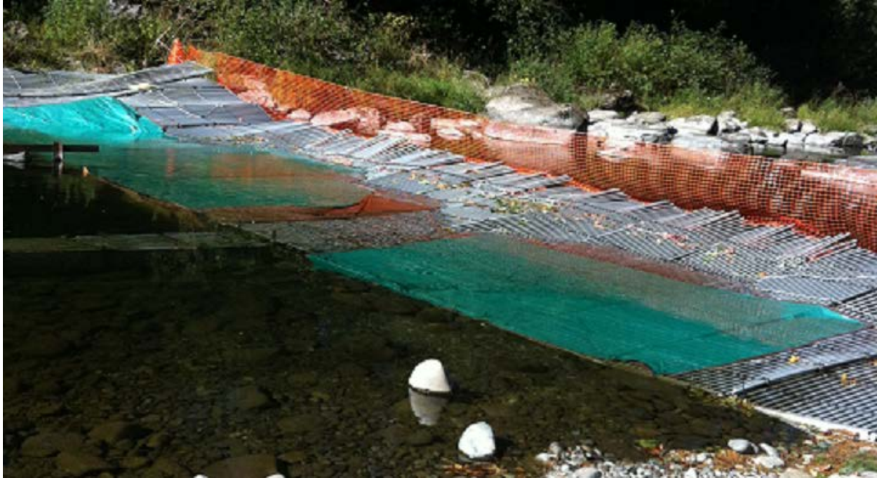
Figure 10. Washougal River Weir configuration, 2012. Photo credit: Jeremy Wilson (WDFW).
