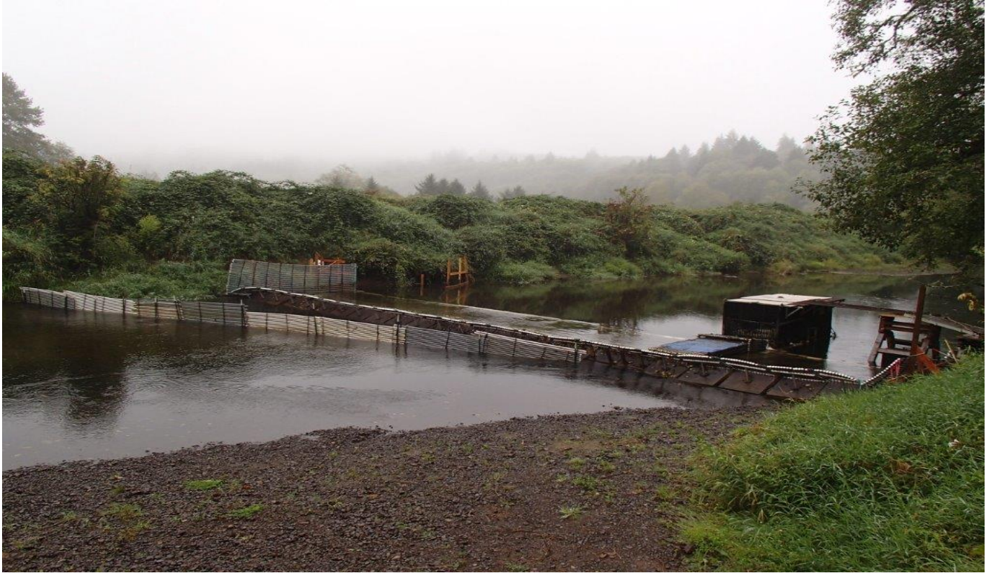
Figure E2. 2016 Grays River Weir configuration.
