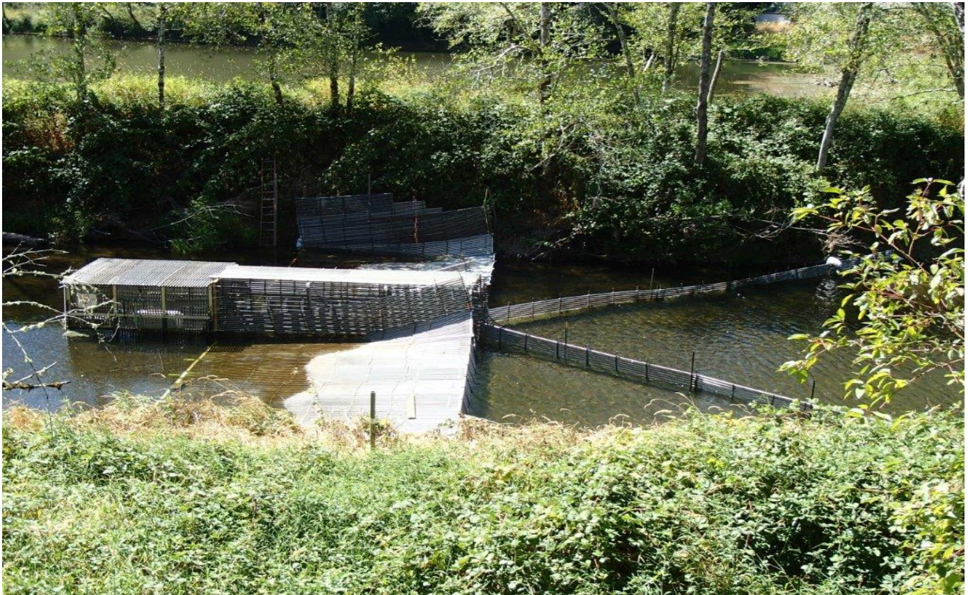
Figure E7. 2017 Coweeman River Weir configuration.
