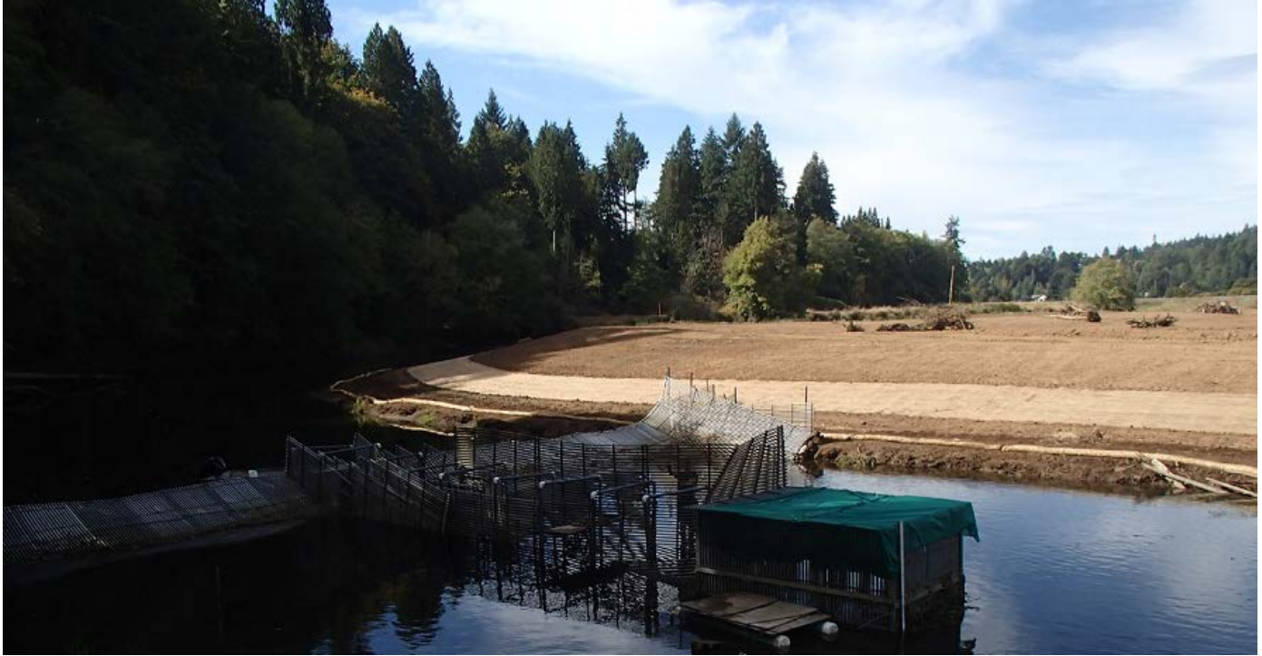
Figure E6. 2016 Coweeman River Weir configuration.
