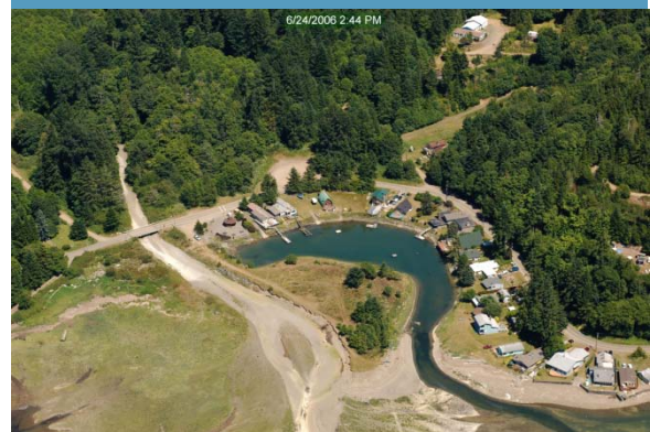
Photo 4-4 Example of embayment that has been partially filled (Photo courtesy of WDOE)
