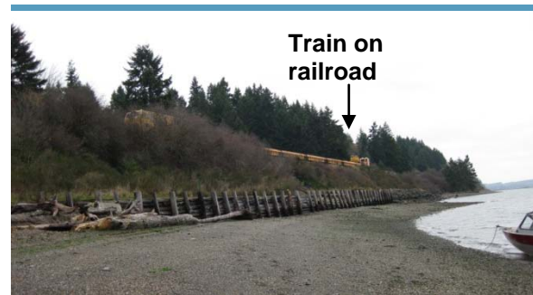
Photo 4-7 Example of railroad along Puget Sound shoreline (Photo courtesy of Anchor QEA)
