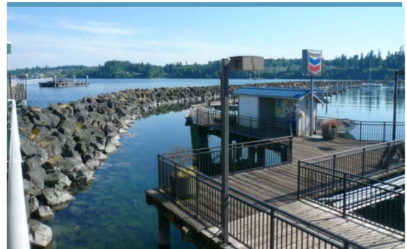
Photo 4-10 Example of jetty along shoreline of Puget Sound (Photo courtesy of Coastal Geologic Services)
