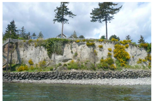
Photo 4-5 Example of shoreline armoring disconnecting a bluff-backed beach (Photo courtesy of Coastal Geologic Services)
