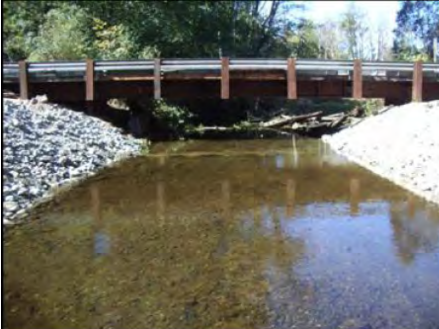
Figure 9-4 Culvert to bridge replacement, Shine Estuary.
