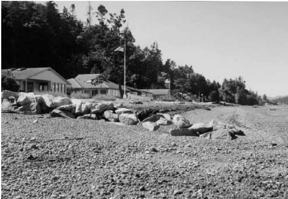
Figure 7-3 Samish Island drift sill that forms the eastern end of nourishment
