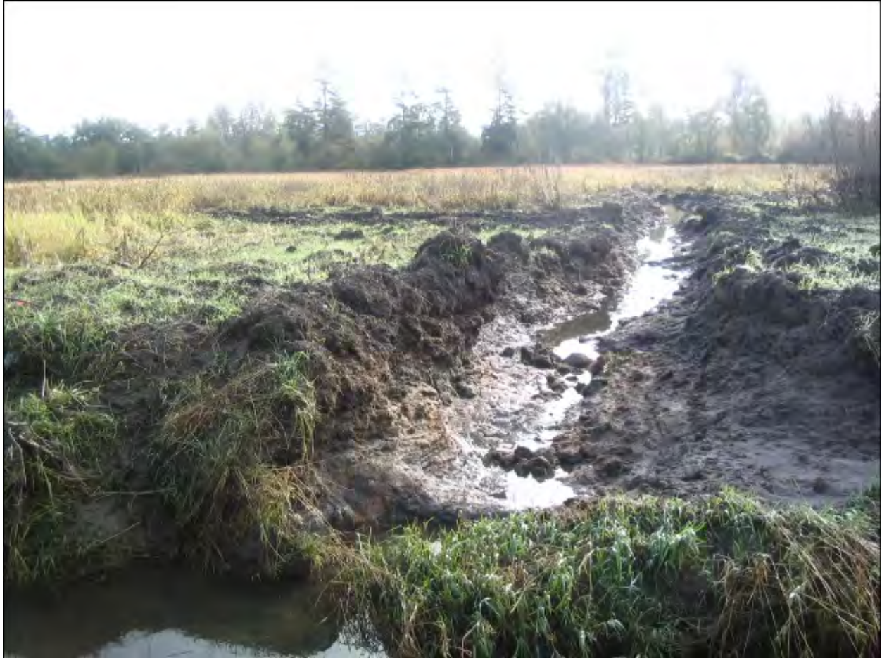
Figure 4-3 Milltown Island tidal channel created with explosives.
