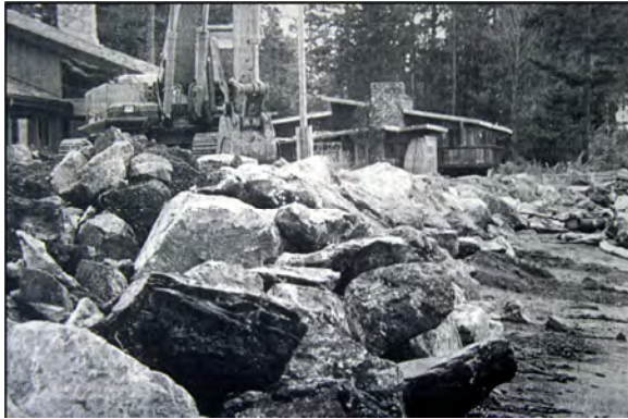
Figure 1-3 North Beach Orcas Island armor removal and beach nourishment: Before (1991) and after (2008) at same location. Before photo by Jan Kolton, after by Jim Johannessen.
