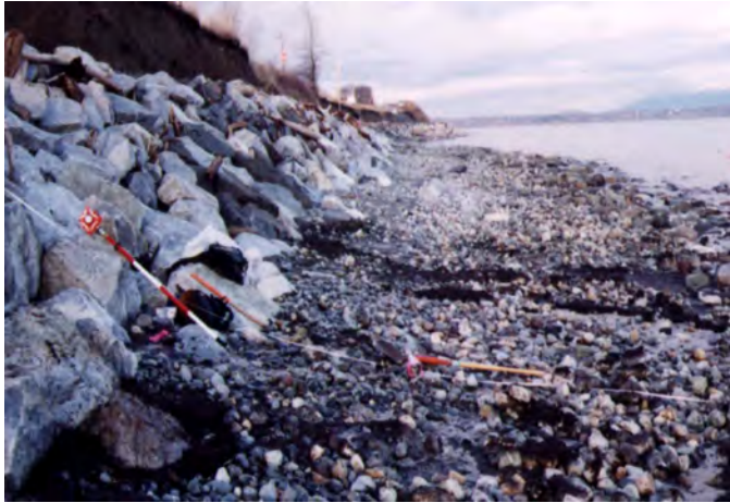
Figure 2-4. Lummi Shore Road, Bellingham Bay beach nourishment: Before (1999) and after (2000) at same location. Both photos by Jim Johannessen.
