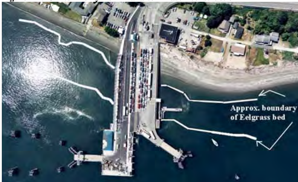
Figure 12-5 Clinton Ferry Terminal after Phase I construction
