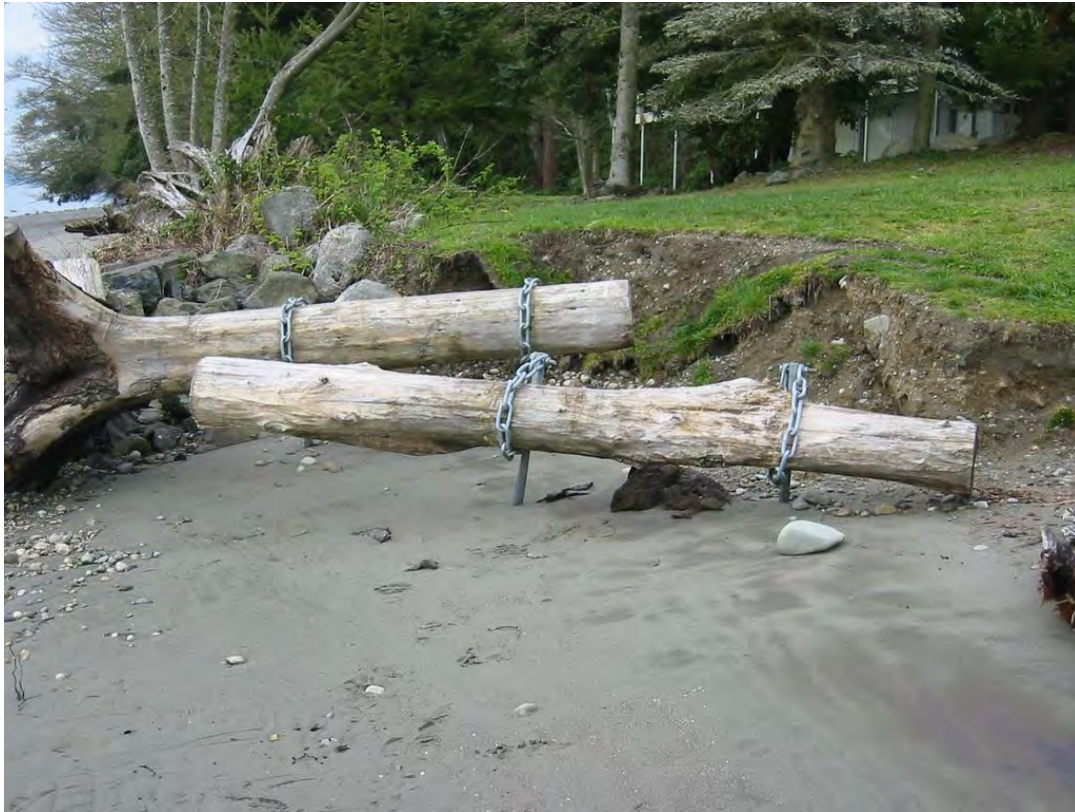
Figure 11-4 Tacoma Narrows Park anchored LWD project in 2006 (Hugh Shipman).
