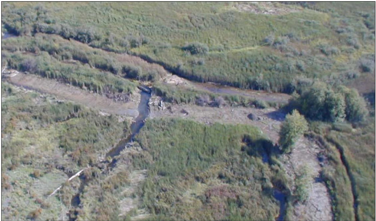
Figure 3-3 Reconnection of remnant channel with outboard channel by excavation through the dike foundation (Hood 2004)
