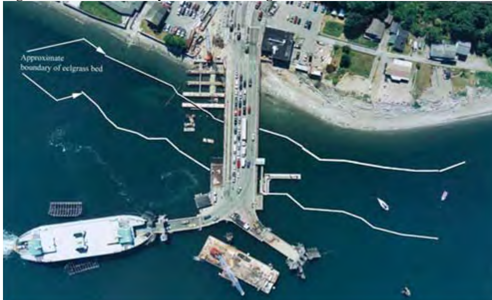
Figure 12-4 Clinton Ferry Terminal during Phase I construction which widened the dock
