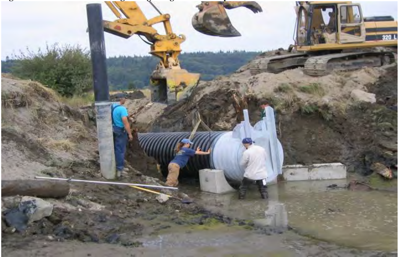
Figure 9-3 Operation of self-regulating tide gate at Fornsby Creek
