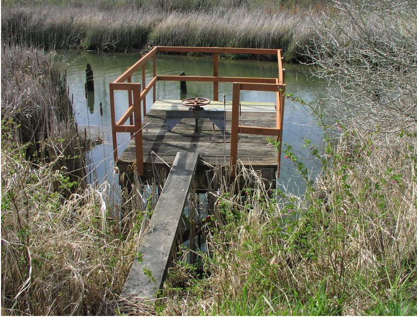
Figure 4. Barn Field water control structures on waterward side of the dike. Footbridge to platform with screw gate controls.
