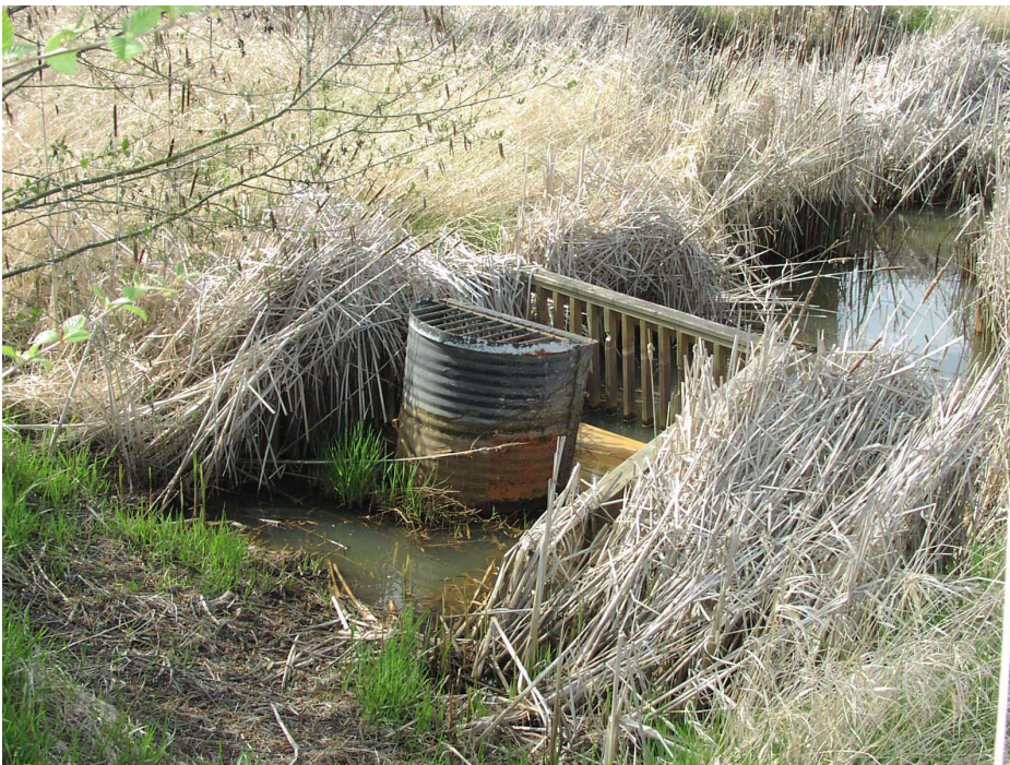
Figure 8. Seattle Pond water control structures on landward side of the dike. Flashboard riser with foot bridge and hand rail.
