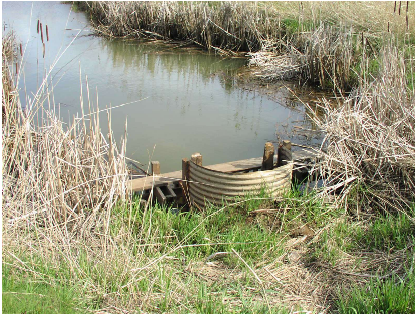
Figure 6. Barn Field water control structures on landward side of the dike. Flashboard riser with foot bridge.
