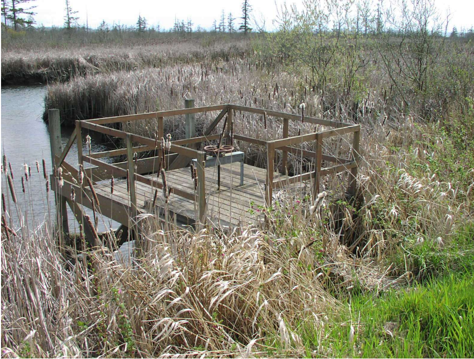
Figure 7. Seattle Pond water control structures on waterward side of the dike. Footbridge to platform with screw gate controls
