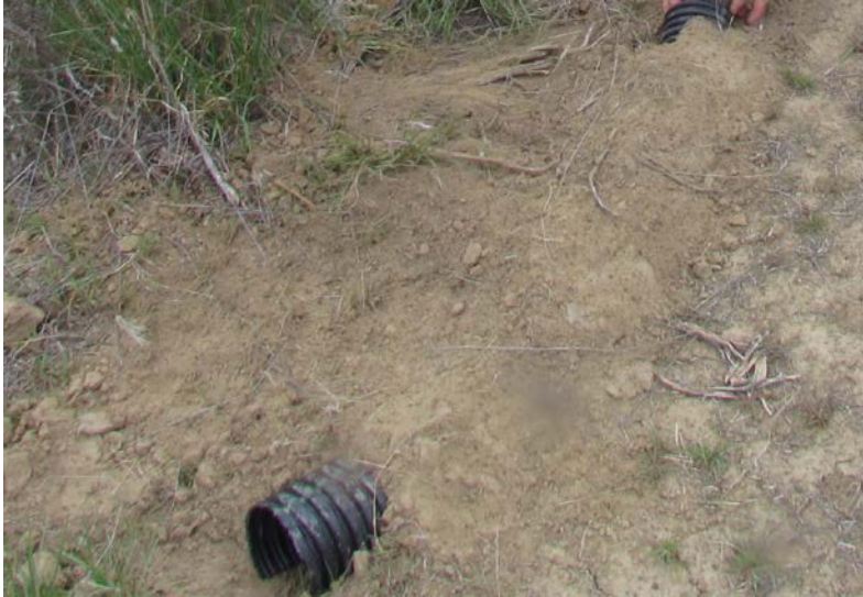
Construction of a hard release site and placement of artificial burrows.
