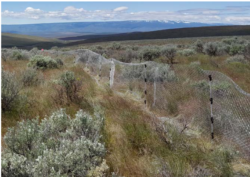
Construction of temporary release pens
