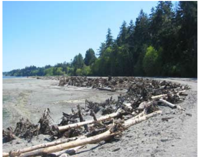
Figure 19. Coastal restoration immediately south of Chiacum Creek mouth, eastern Jefferson County (Hugh Shipman). Large woody debris was placed on the waterward edge of a reduced fill area.
