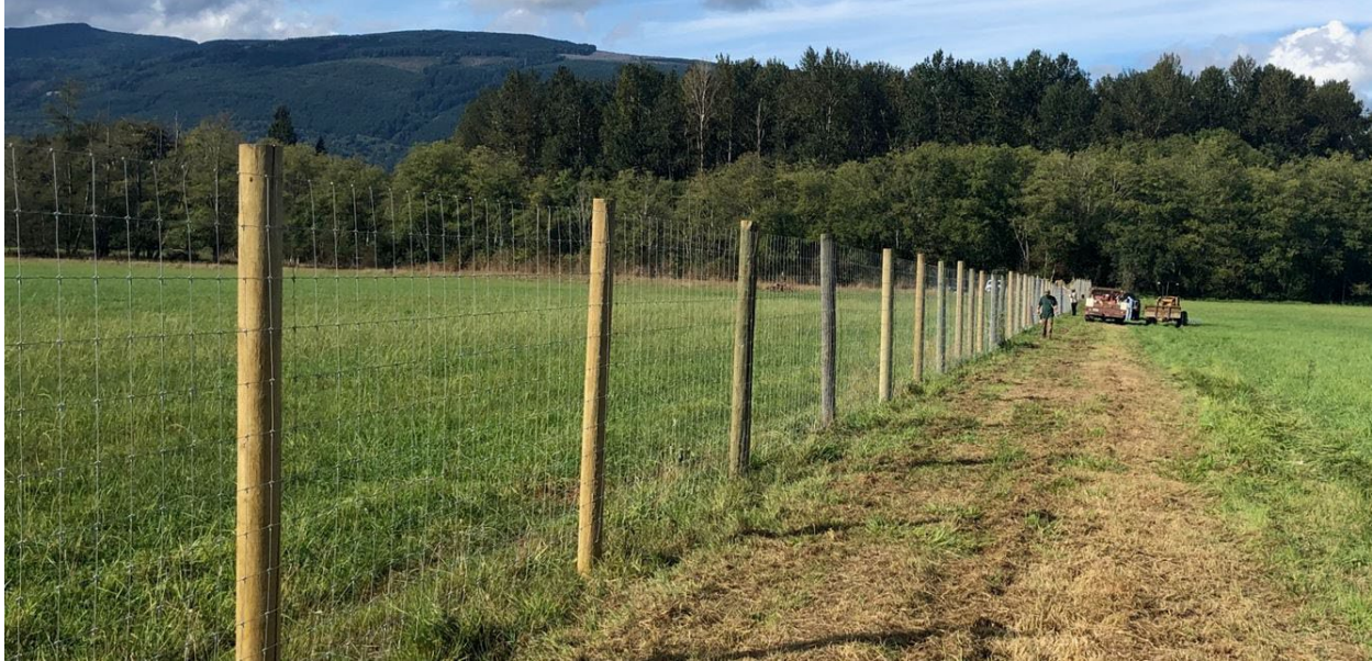
Figure 3. Fencing project in Day Creek
