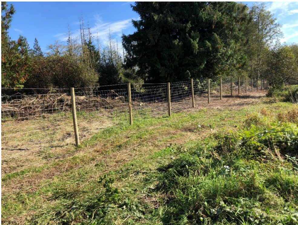
Figure 2. Completed woven wire fencing on property adjacent to SR20. To date, no elk intrusions have occurred on the property since installation of the fence.
