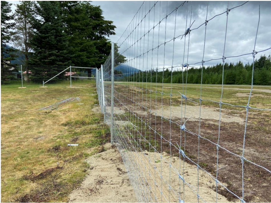
Detail of the New Zealand style fence installed along the school's perimeter.
