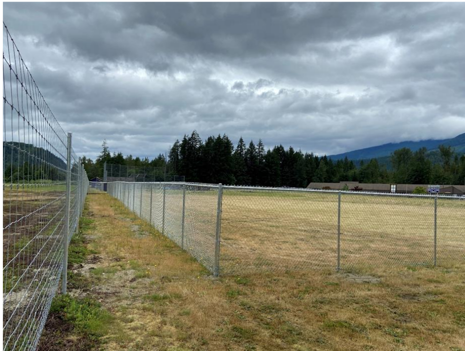
Photo detailing the two types of elk fencing installed by the Concrete School District. At this location, New Zealand style fencing extends along the school's southern boundary with the Concrete Municipal Airport, and chain link fencing surrounds the baseball field.
