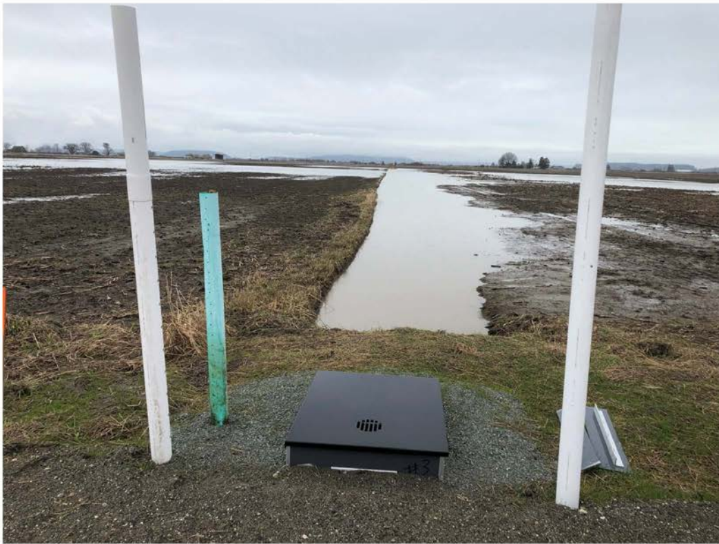
FIGURE 6 Water control structure managing water in working farmlands (holding water).
