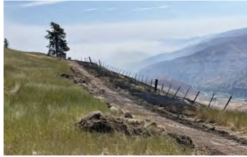
Figures 11 & 12: Establishing a fire break in some areas assist in the containment efforts. Unfortunately, the Department will need to replace about 6 miles of boundary fence along neighboring properties as well as interior fence. Department staff are still assessing the damaged interior fence and cost estimates for interior fence replacement are not identified in this request until more information is available. Photo credit, Bob Dice, Chief Joseph Wildlife Area Manager
