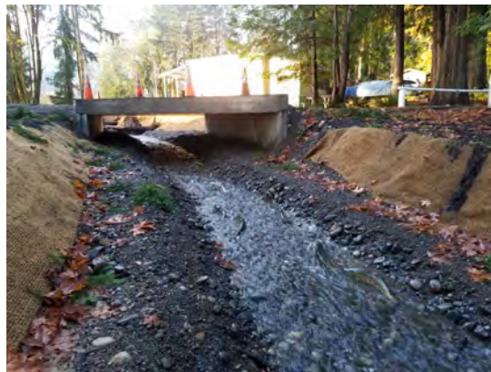
Completion of fish passage restoration project at Potlatch State Park.
