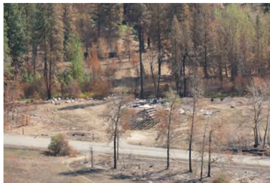
684 Eastside Chewuch Rd. Winthrop, WA 98862 - Dammann Dairy barns impacted in the Cub Creek 2 fire. The barn in the forefront survived the fire, but the 1920's barn behind, fully consumed in the fire, will require labor-intensive cleanup. (Photo courtesy of Methow Wildlife Area Manager, Brandon Troyer.)
